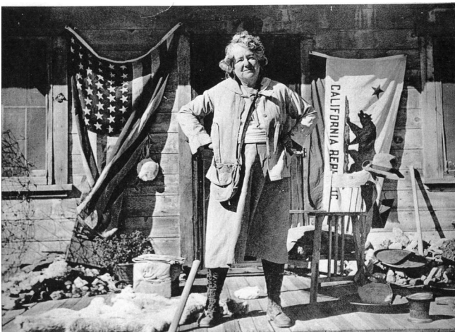
Josie on Front Porch of Main Cabin
